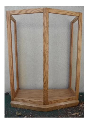
**Ron Gerard** Described the start of the curio cabinet he's making from oak. To keep the cabinet from looking like a rectangular box, the face is angled out with two doors on each face that is yet to be made. For the first time, he has prefinished the parts with wipe-on polyurethane. Seven coats were applied on the horizontal portion of the base and five coats elsewhere. An additional coat of Maloof's oil and wax finish covers all surfaces.
