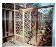
A portion of the fence has 6 X 6 concrete wire attached to the fence frame with thin redwood strips woven through the wire. The concrete wire sticks up beyond the top of
