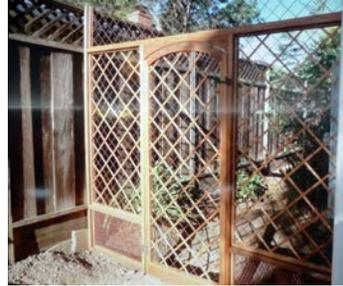
A portion of the fence has 6 X 6 concrete wire attached to the fence frame with thin redwood strips woven through the wire. The concrete wire sticks up beyond the top of the fence and is cut to form spikes at the top so as to keep cats and raccoons from walking on the fence and jumping on the roof.
