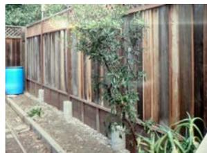
than her yard, concrete pillars are sunk into the ground to a depth of about three feet that extend above the ground about 18 inches. When digging a hole to that depth, it is difficult to clean out the dirt at the bottom. Tracie used a novel approach by using a shop vacuum to clean out the dirt!
